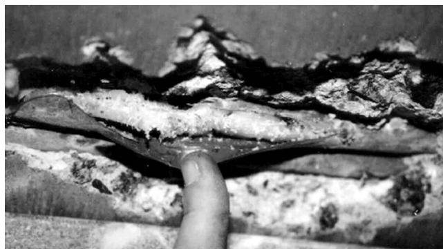
Fig. 6.2—Cured urethane grout completely encapsulating a monostrand tendon.
