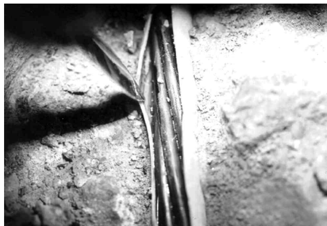
Fig. 5.3—In-place examination of an unbonded tendon.
