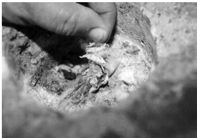
Fig. 5.2—Existing damage to tendon duct.
