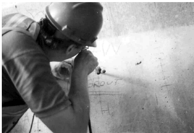
Fig. 5.6—Field examination of grouted tendon duct with invasive probing.
