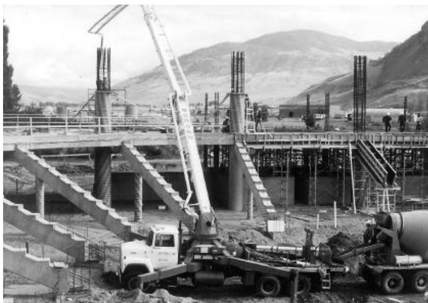
Fig. 7—Truck engine-driven concrete pump
