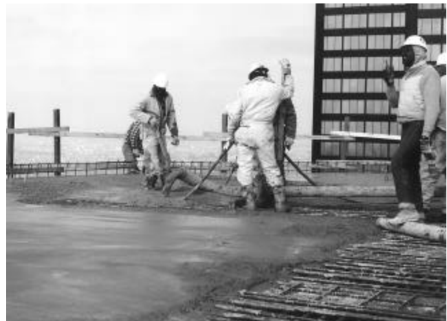
Fig. 15—Spreading concrete with flexible hose at the end of a rigid pipeline
