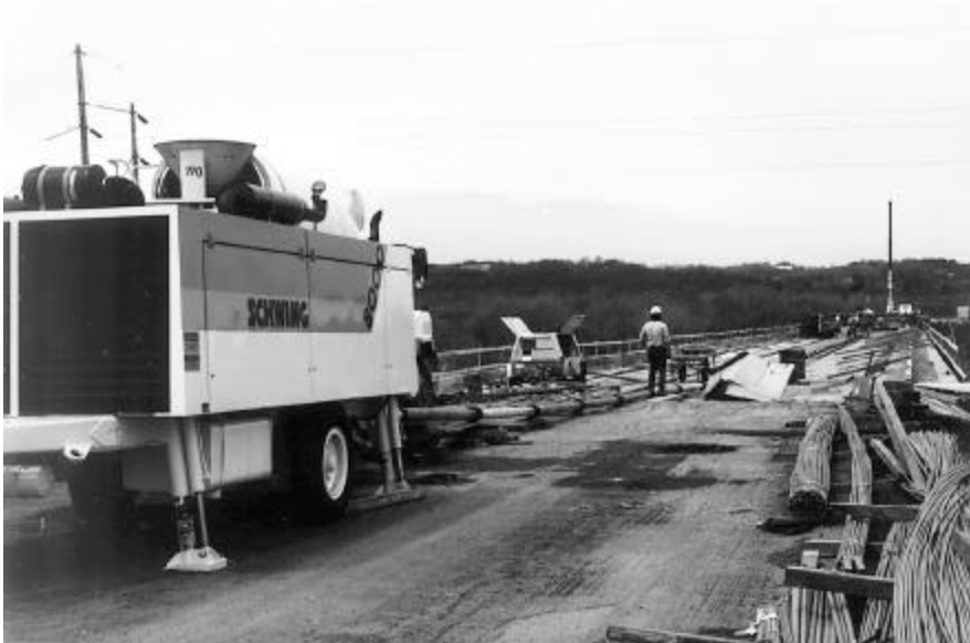
Fig. 6—Special application-type trailer-mounted concrete pump
