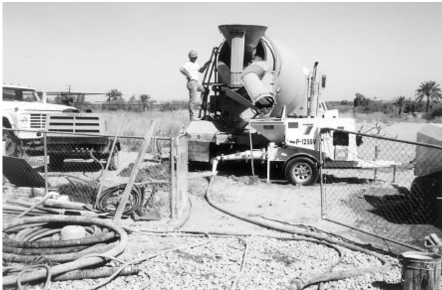
Fig. 3—Ball check concrete pump
