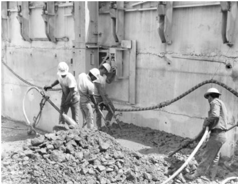
Fig. 9.4(b)—Flattening a pile of mass concrete just deposited in form
