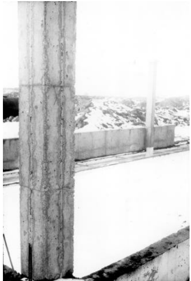
Fig. 6.4—Sand streaks caused by mortar leak
