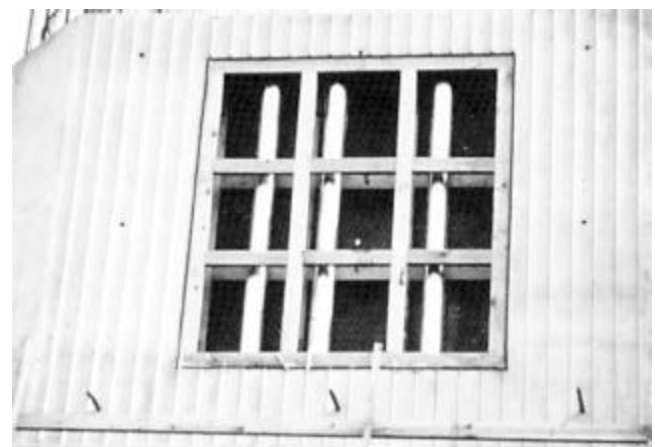
Fig. 17.1.3—Large blackout within a wall with pipes through the formed blackout to permit access for concrete placement and vibration
