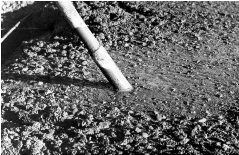
Fig. 4—Internal vibrator “liquifying” low-slump concrete
