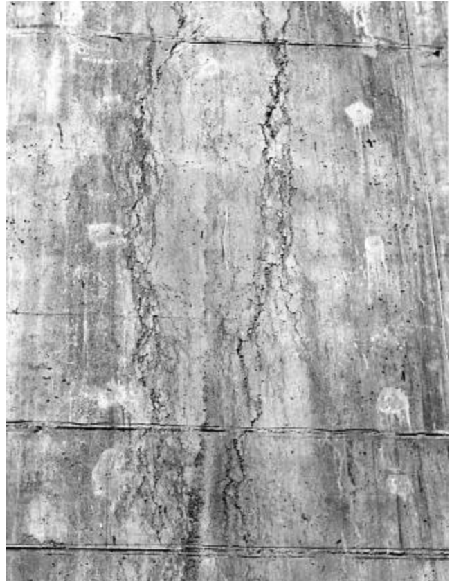
Fig. 7.6.3—Sand streaking caused by heavy bleeding along form
