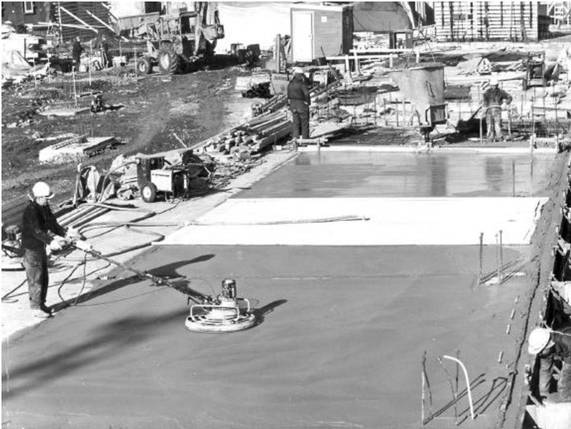
Fig. 10.6—Vacuum dewatering of concrete slab is shown just behind the floor finishing operation
