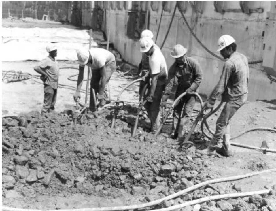
Fig. 9.4(c)—Systematic vibration of concrete layer
