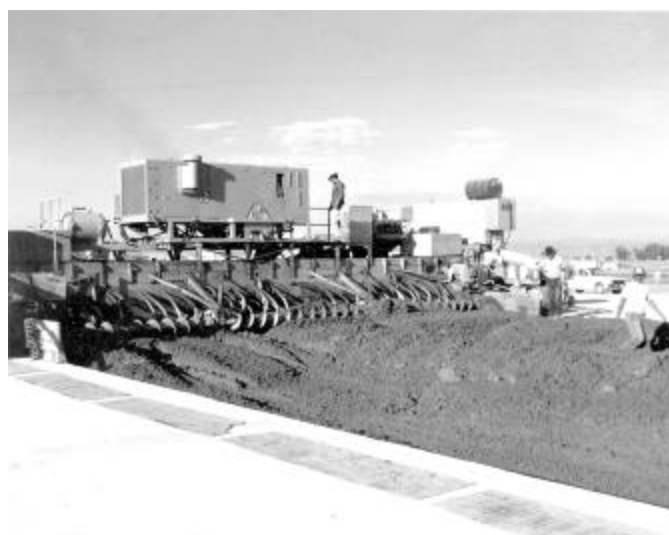
Fig. 11.2.4(b)—Older screeds with trucks permitting cam-like action to raise screed to clear concrete surface when moving for second pass
