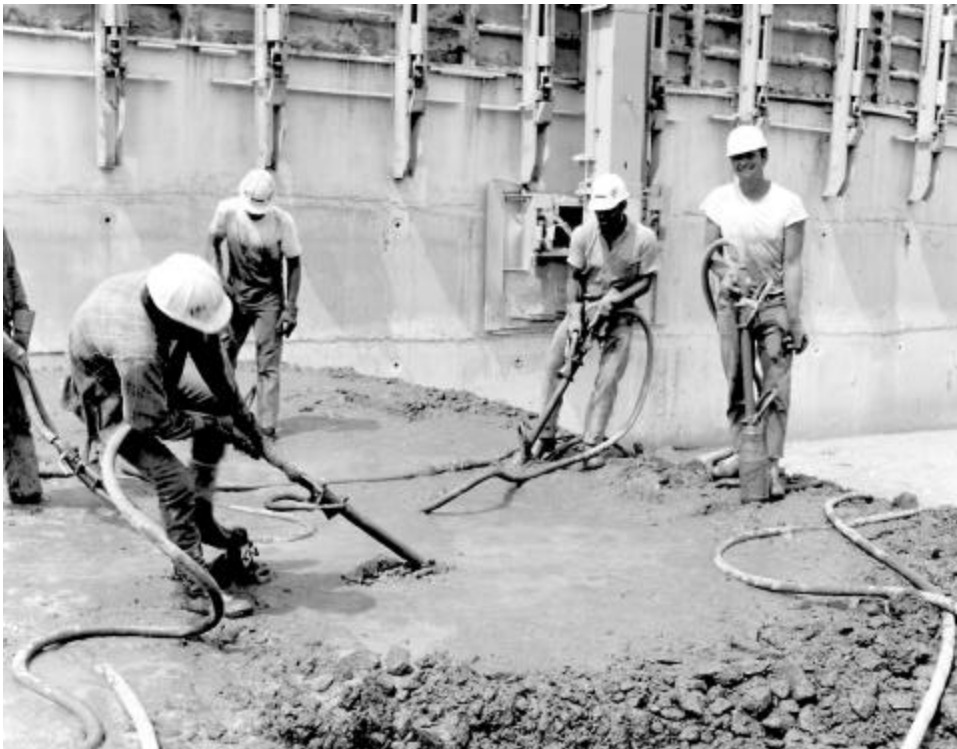
Fig. 7.6.1(b)—Haphazard procedure may result in mortar accumulation at the surface and leave rock pockets below, particularly at batch perimeters
