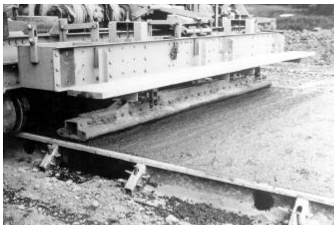
Fig. 11.2.4(a)—Pan-type surface vibrator for pavement construction
