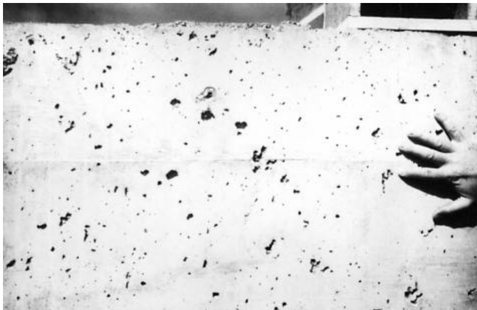
Fig. 7.6.2—Excessive air voids on formed surface
