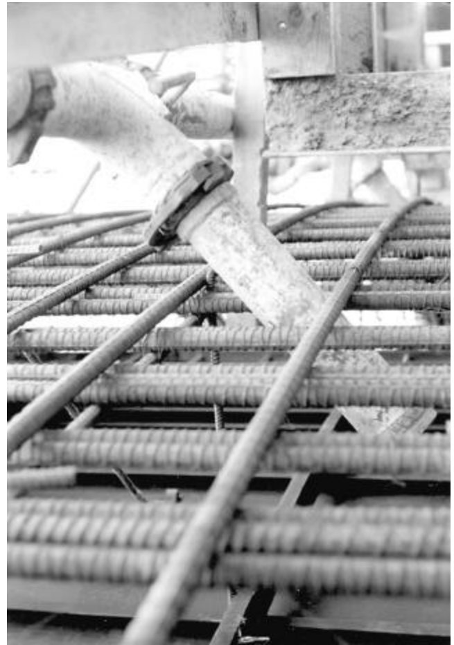
Fig. 17.1.2—Congestion due to a pipe passing through a concrete floor
