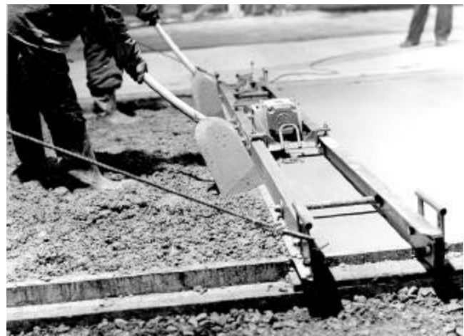
Fig. 5.4(b)—Vibrating screed for small jobs. Double beam type
