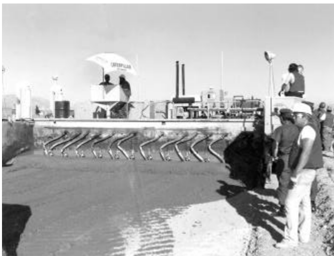
Fig. 11.2.3—Gang-mounted spud vibrators for consolidating pavement concrete
