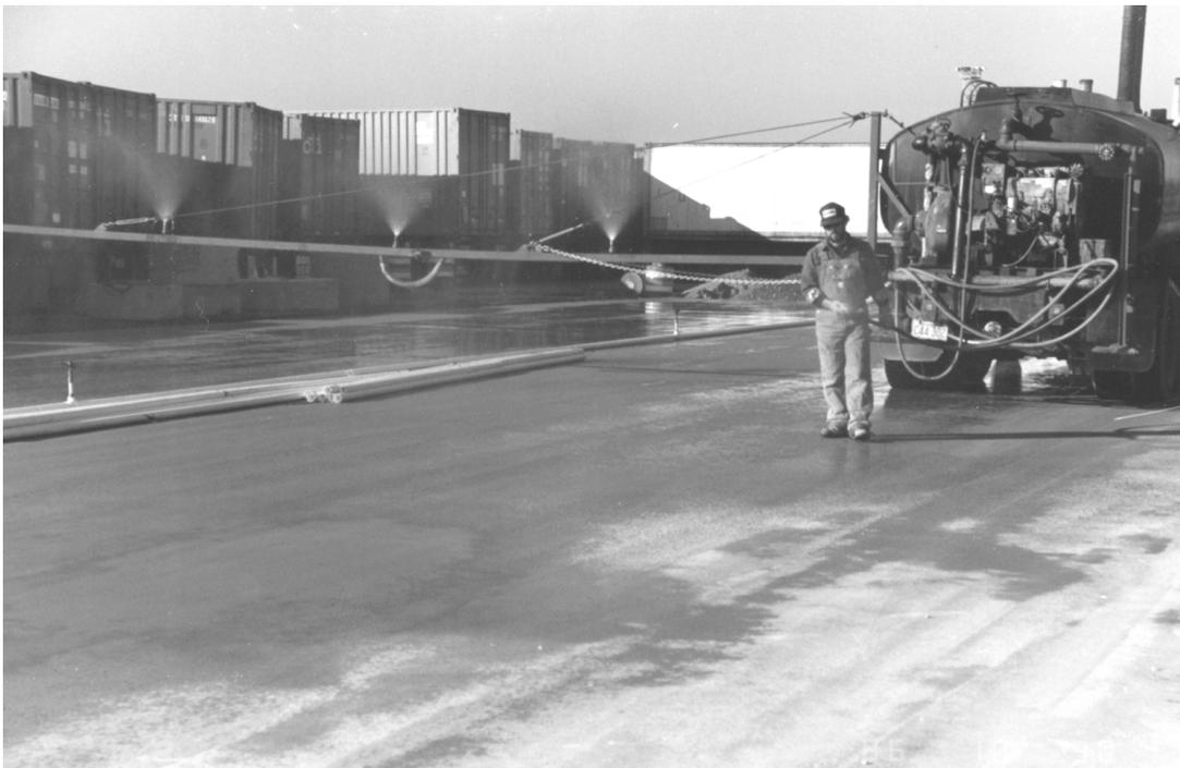
*Fig. 2.4—Fog curing of freshly placed RCC pavement*
