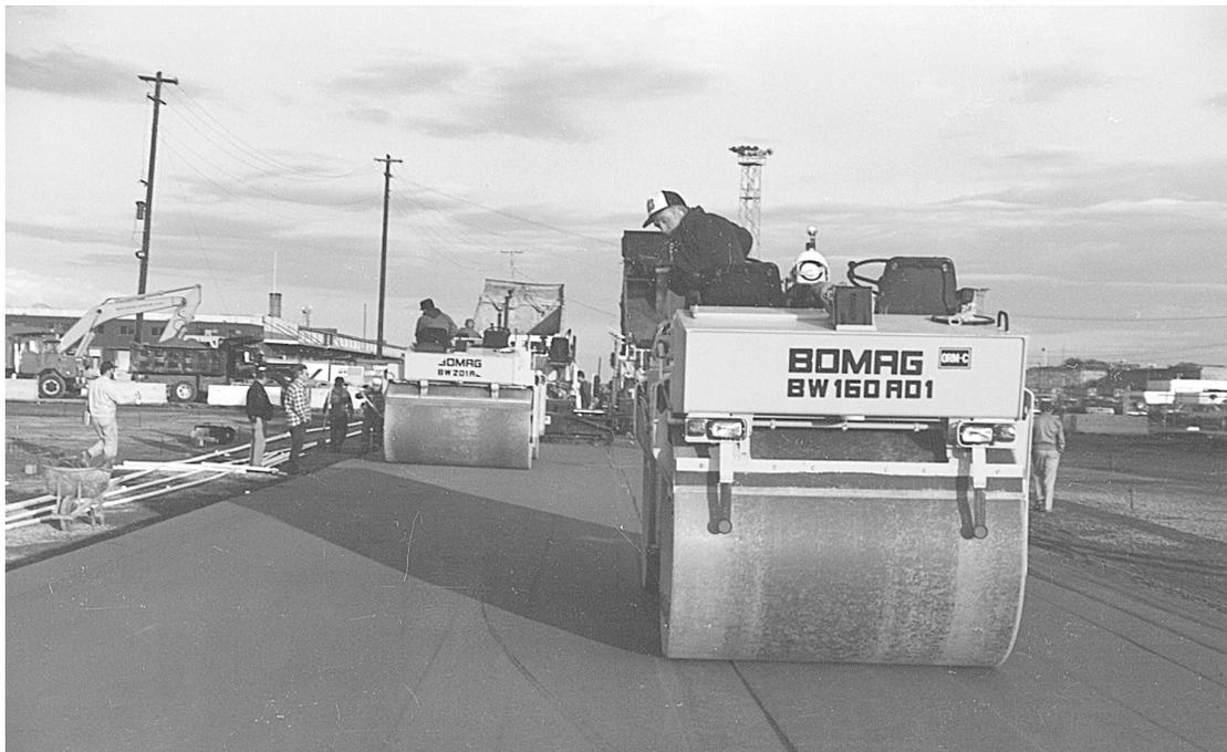
*Fig. 2.2—Vibratory roller compaction*
