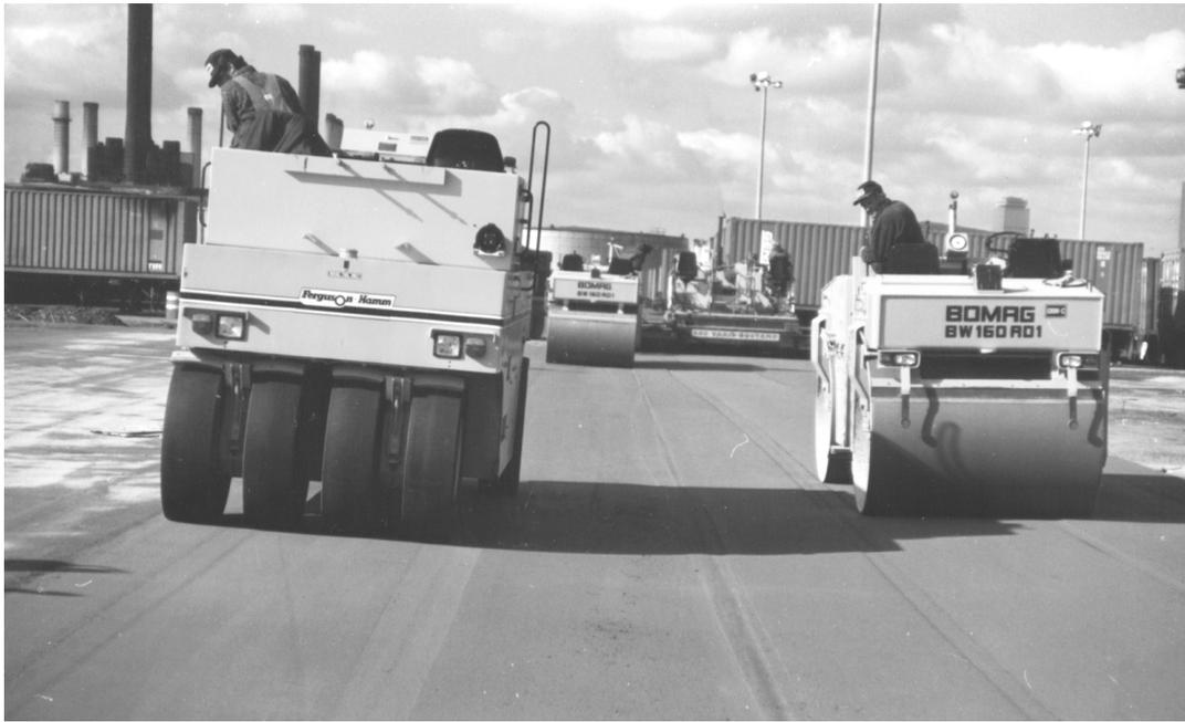
*Fig. 2.3—Rubber-tired roller compaction*
