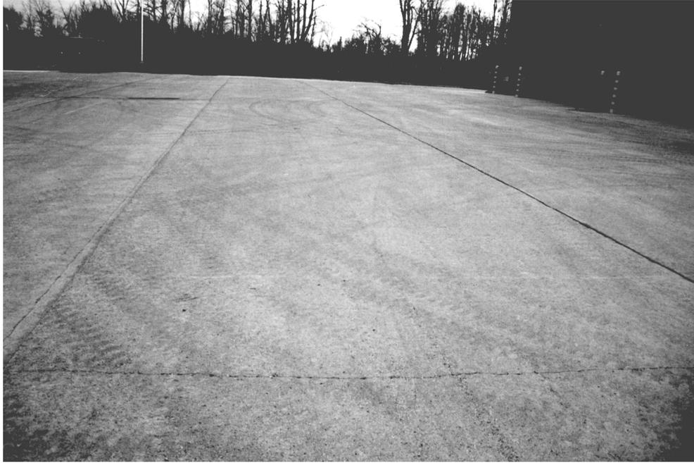
*Fig. 2.5—RCC pavement — Ft. Drum, New York*
