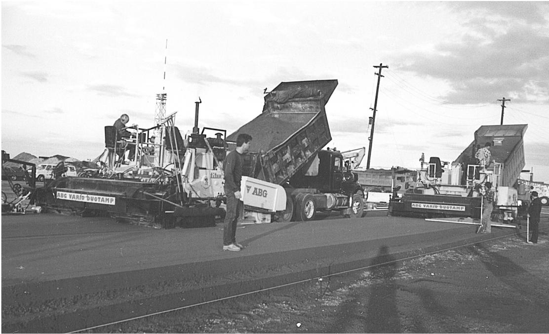
*Fig. 2.1—RCC placement using modified asphalt pavers*
