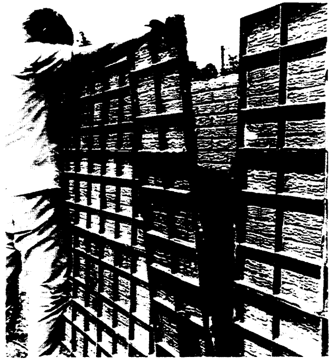
Fig. 5.1 (b)--Manufactured all-aluminum forms. This set produces brick texture
