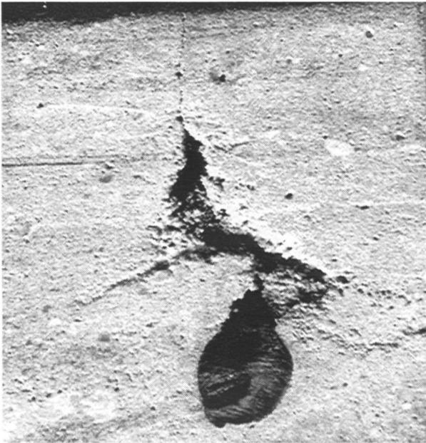
*Fig. 4.1-Serious sandpocket developed because of carelessness of nozzle men. Use of the No. 6 bar made proper encasement more difficult but with careful and skilled nozzling, the work could have been properly accomplished. Note the fine crack above the bar and also mending down from the bottom of the sandpocket. When cracking develops above the line of a bar, a continuous sandpocket may be suspected behind the bar. The sandpocket reduces the section area, encouraging cracking.*
