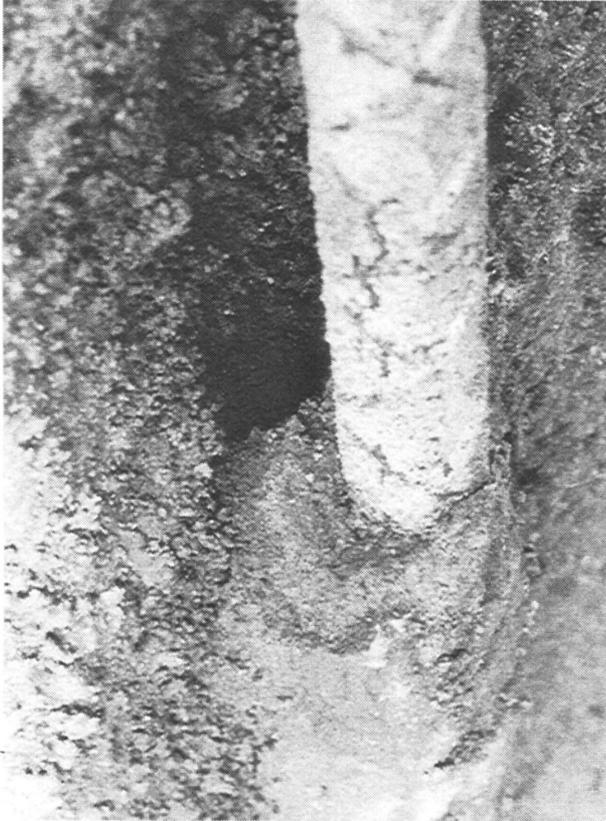
Fig. 4.3 void behind bar caused by failure to remove overspray
