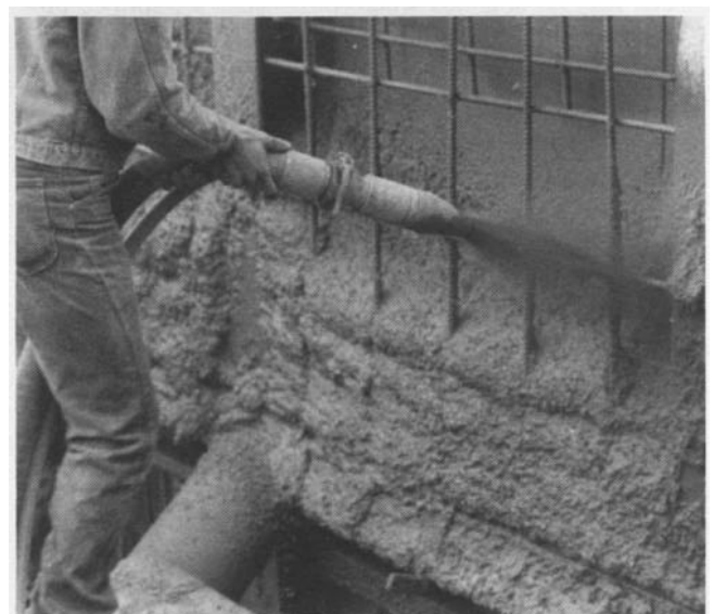
Fig. 8.3-Wet gunning around reinforcing bars. Shotcrete is 11 in. (280 mm) thick
