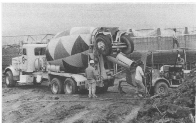
Fig. 3.10-Ready-mixed concrete truck delivering material to wet-mix shotcrete pump
