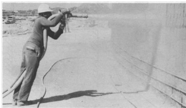
Fig. 8.1b-Correct gunning position-Nozzle perpendicular to receiving surface
