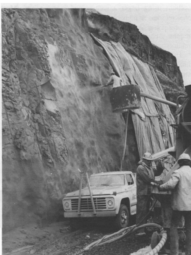
Fig. 1.4-Applying steel fiber reinforced dry-mix shotcrete against a rock embankment to stabilize the slope. Note that welded wire fabric is not required
