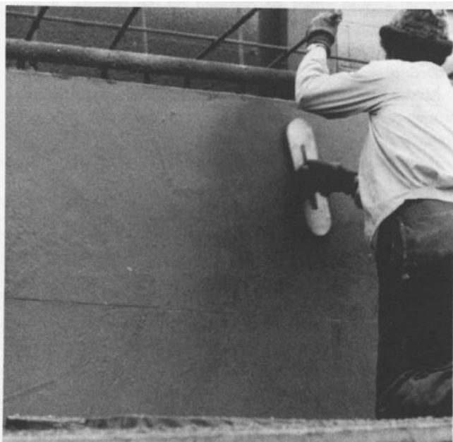
Fig. 8.13a—Applying a steel trowel finish to freshly gunned shotcrete surface
