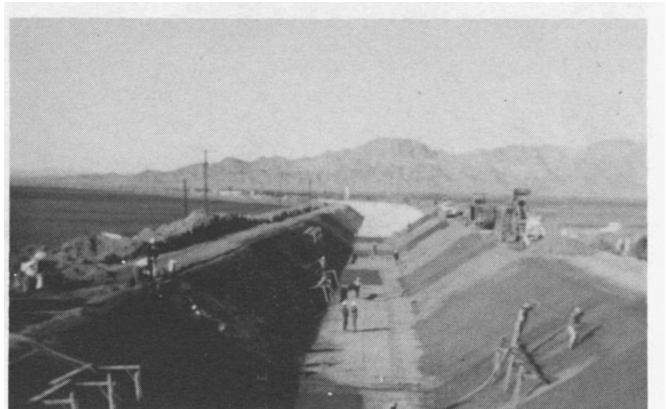
Fig. 1.2-Dry-mix shotcrete lining being installed in a large water irrigation channel in Arizona
