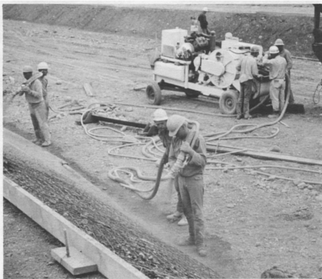
Fig. 1.3a-Applying wet-mix shotcrete as scour protection to a spawning channel
