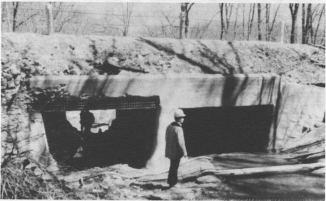
Fig. 1.5b-Concrete in culvert partially restored with shotcrete with a "natural" or gun finish. Final lines are uneven to match the environment, and also reduce finishing costs
