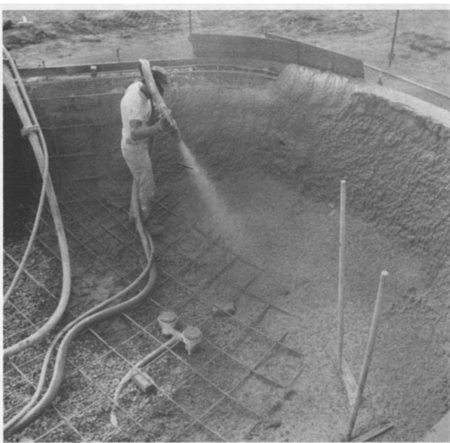
Fig. 1.3b-Applying wet-mix shotcrete in a swimming pool
