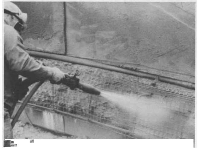
Fig. 5.2-Gunning through welded wire fabric cut and bent to follow contours of repair
