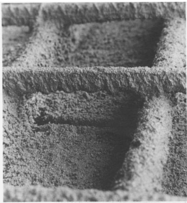
Fig. 8.11-Overspray on reinforcing bars at the top of a band of shotcrete. If the overspray is permitted to harden, and remain on the bars during the next application of shotcrete it will be impossible to fill behind the bars with good shotcrete. Large hollows will remain within the wall, promoting cracking and moisture penetration.
