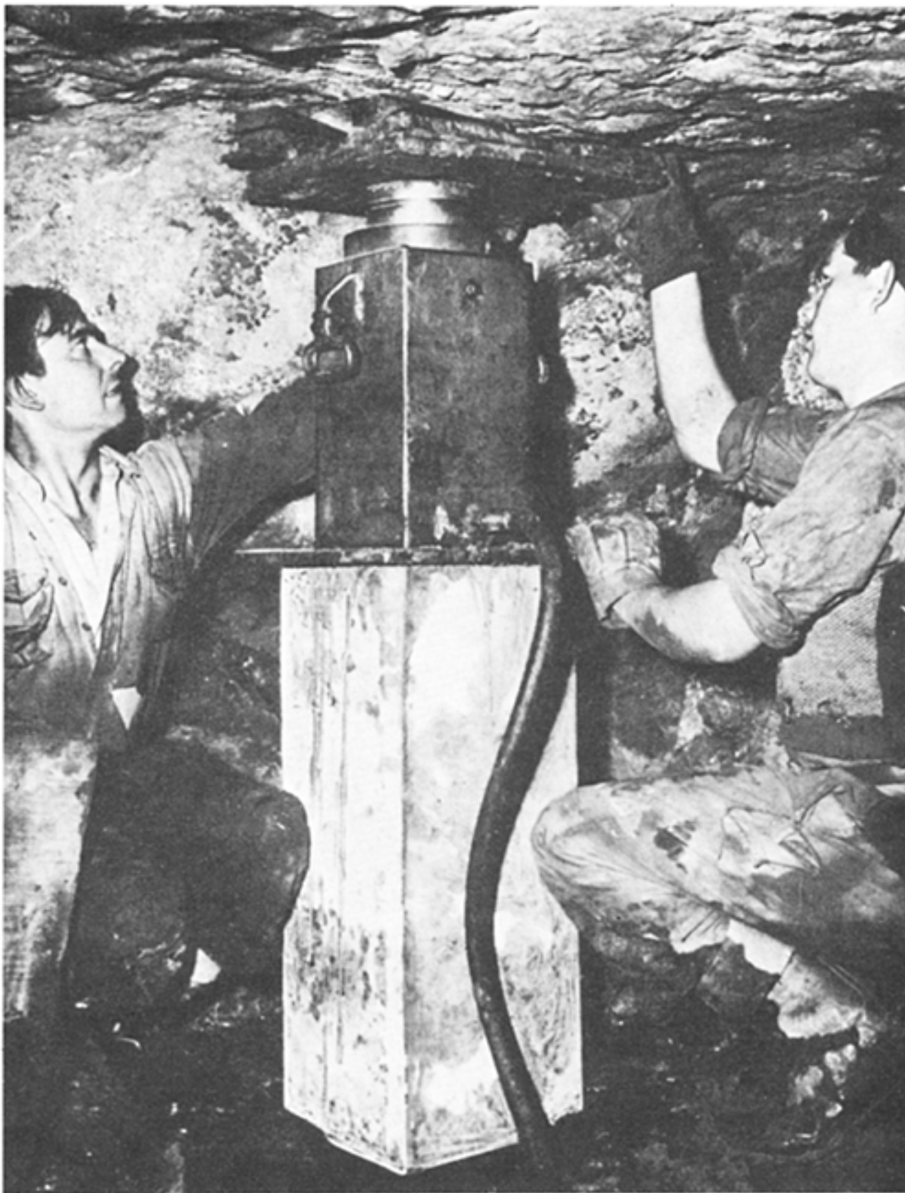
Fig. 9.6 Jacking down Franki Miga pile
