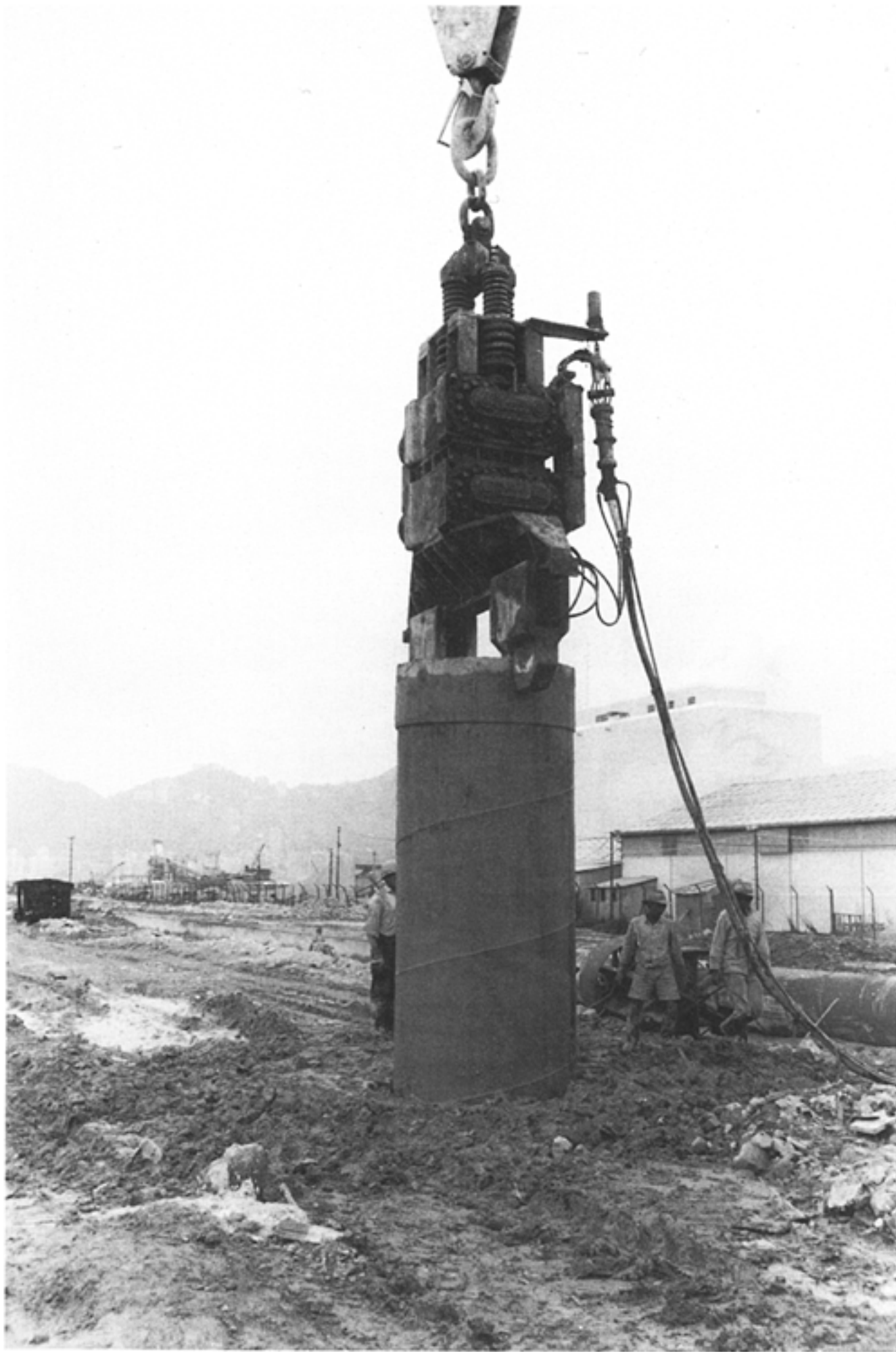
Fig. 3.17 Driving pile casing with Muller vibrator.
