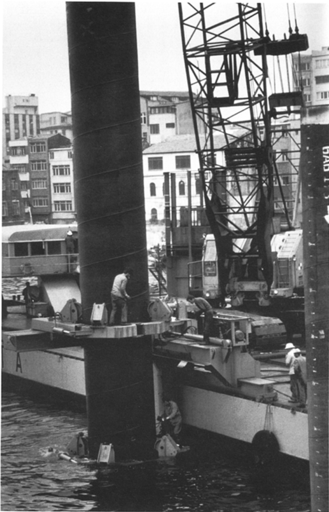
Fig. 3.8 Barge-mounted pile guides with hydraulically-operated clamps
