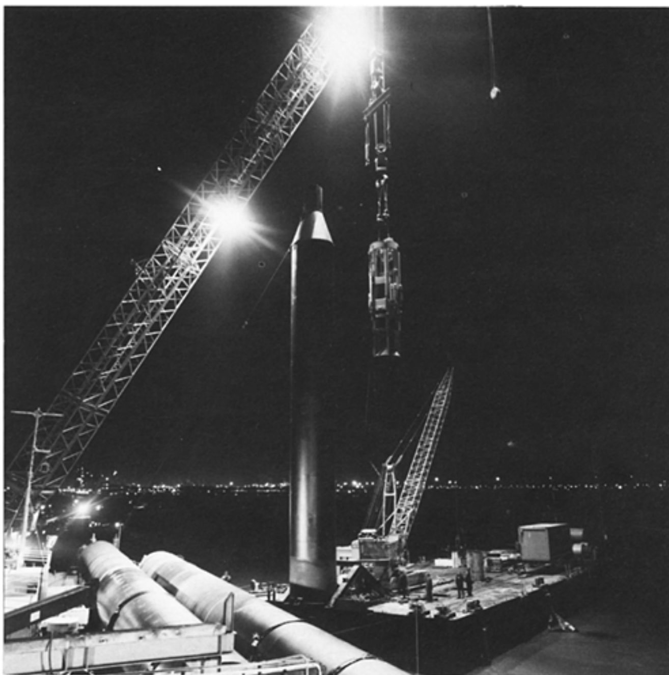
Fig. 3.15 BSP International Foundations Ltd. 40-tonne hydraulic hammer
