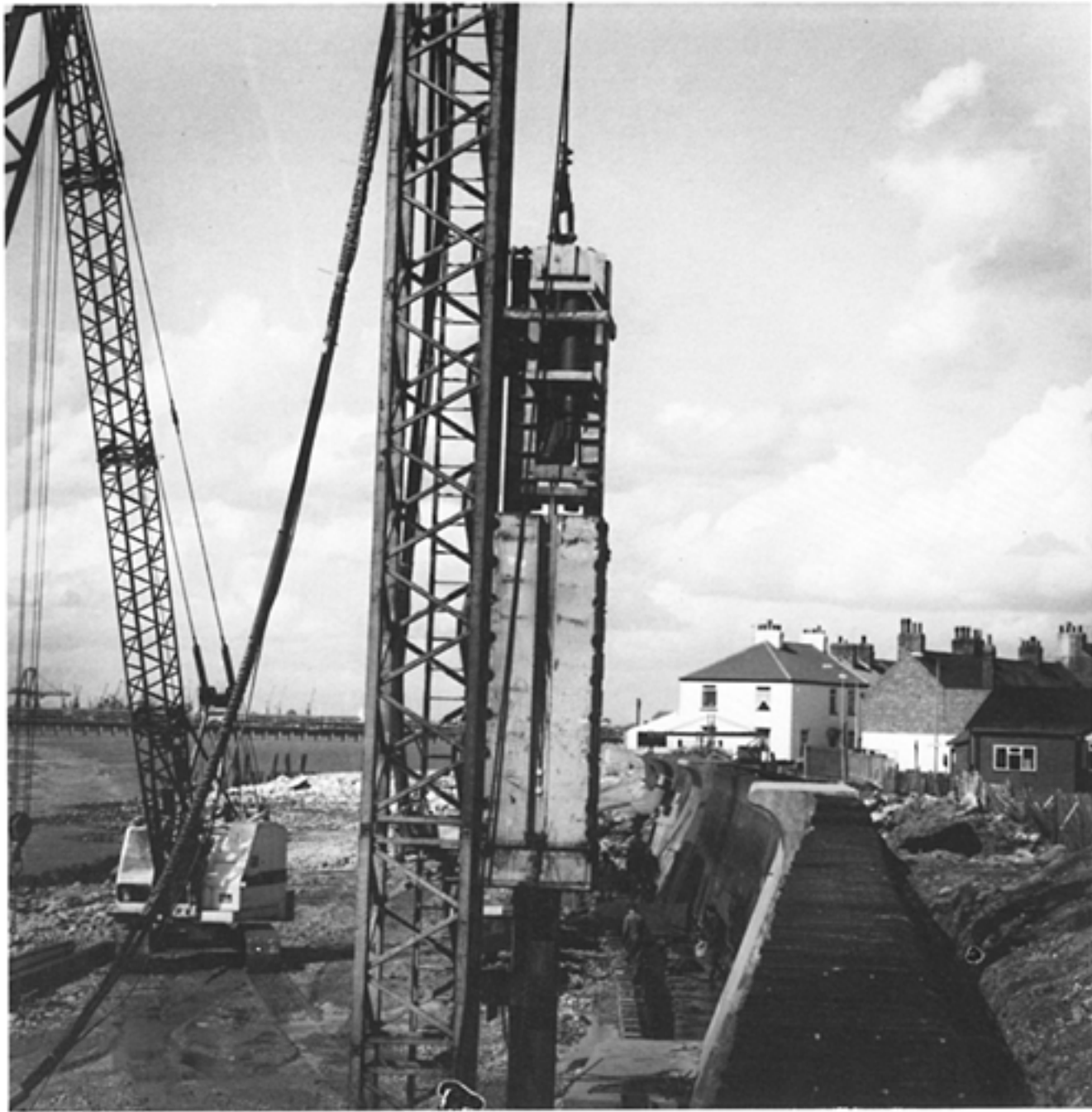
Fig. 3.14 BSP International Foundations Ltd. hydraulic piling hammer
