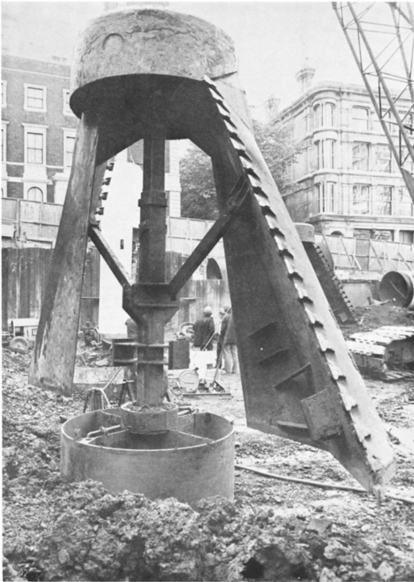
Fig. 3.30 Top-hinged under-reaming bucket
