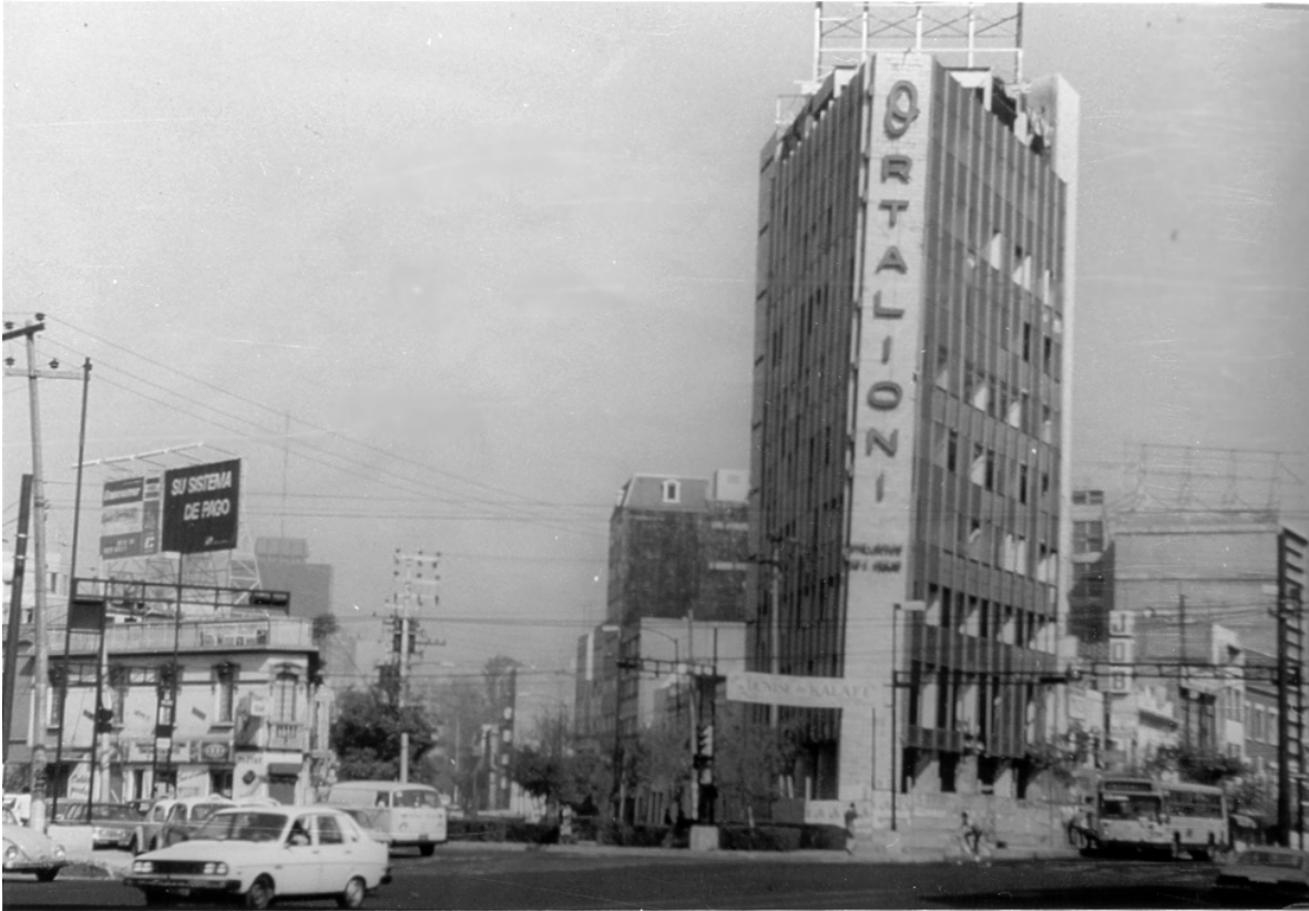
Figure 6-25. Distortion in wedge-shaped building, Mexico City, 1985
