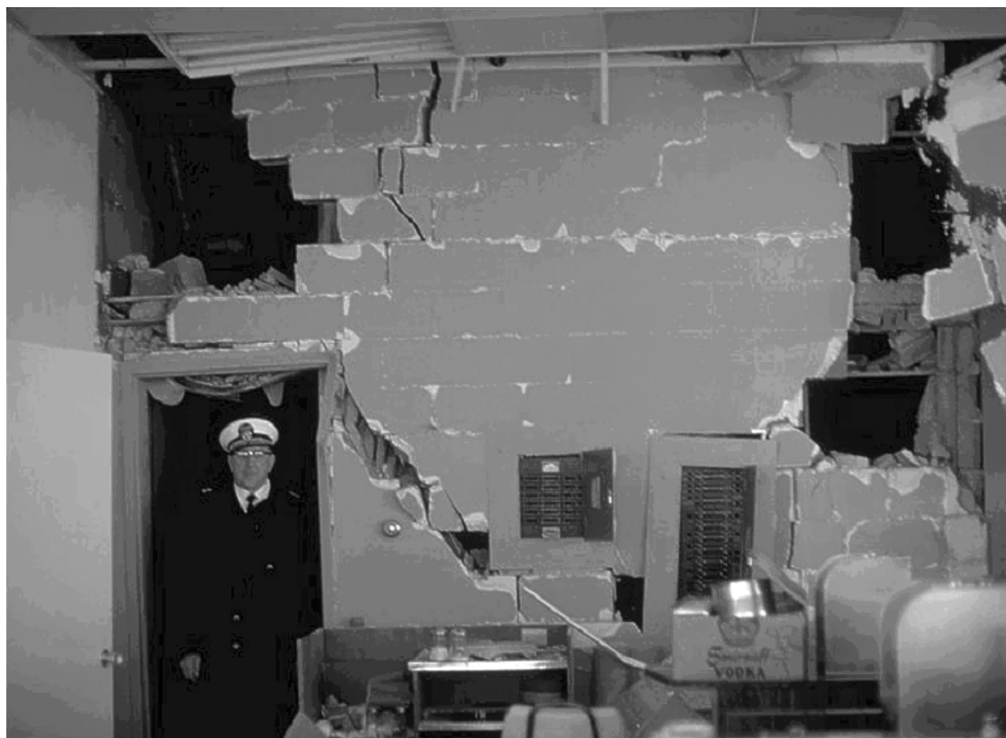
Figure 13-5. Nonstructural partition acting as a shear wall, 1964 Alaskan Earthquake. (Steinbrugge Collection, Earthquake Engineering Research Center, University of California, Berkeley.)
