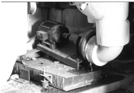
Figure 13-4. Failure of a flexibly mounted pump connected to a braced piping system, 1994 Northridge Earthquake
