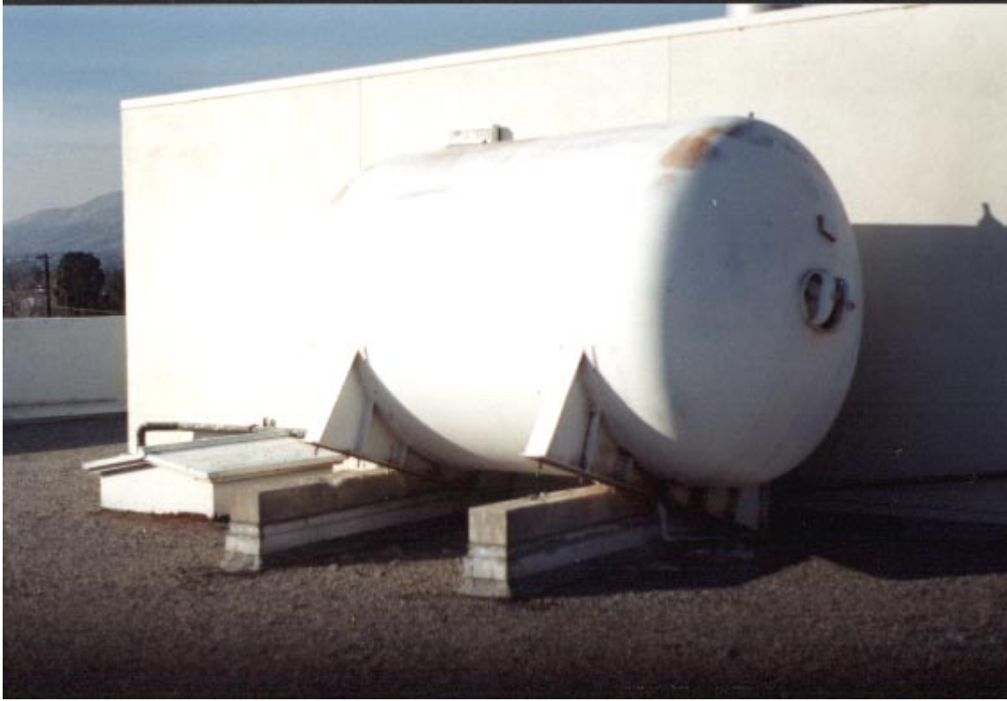
Figure 13-2. Rooftop tank failure, 1994 Northridge Earthquake
