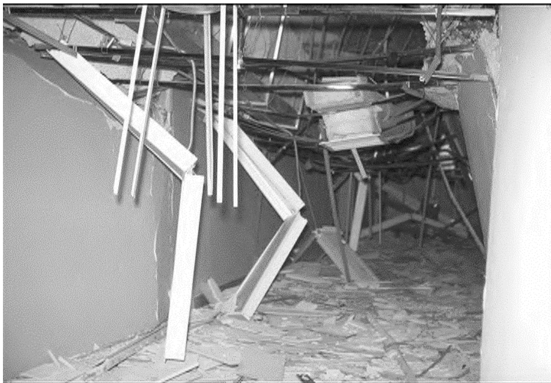
Figure 13-1. Damaged suspended ceiling and light fixtures, Olive View Hospital, San Fernando Valley Earthquake of 1971 (Steinbrugge Collection, Earthquake Engineering Research Center, University of California, Berkeley.)
